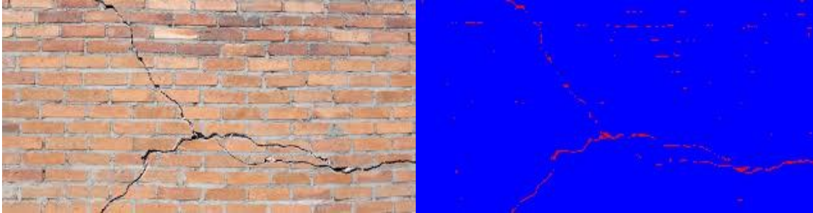
Figure 2: An example of cracks data and segmented cracks
